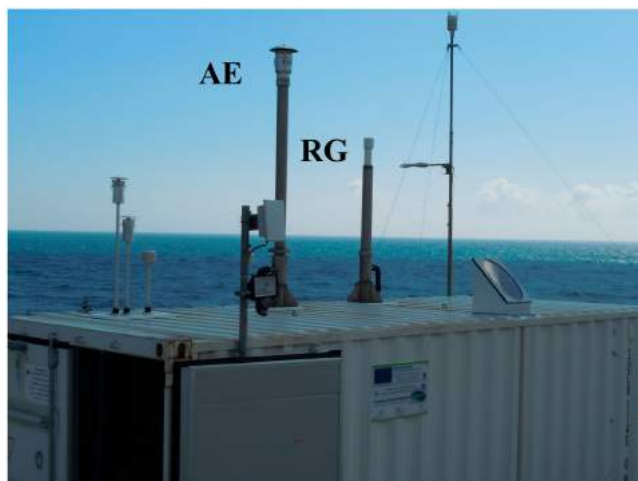
Figure 4. External view of the WMO/GAW regional station at Capo Granitola (CGR): AE and RG sampling systems are indicated.
